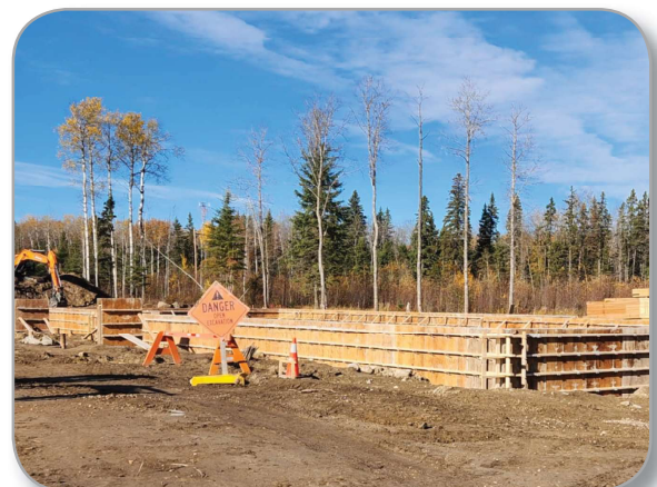
WOMEN'S SHELTER CONSTRUCTION
